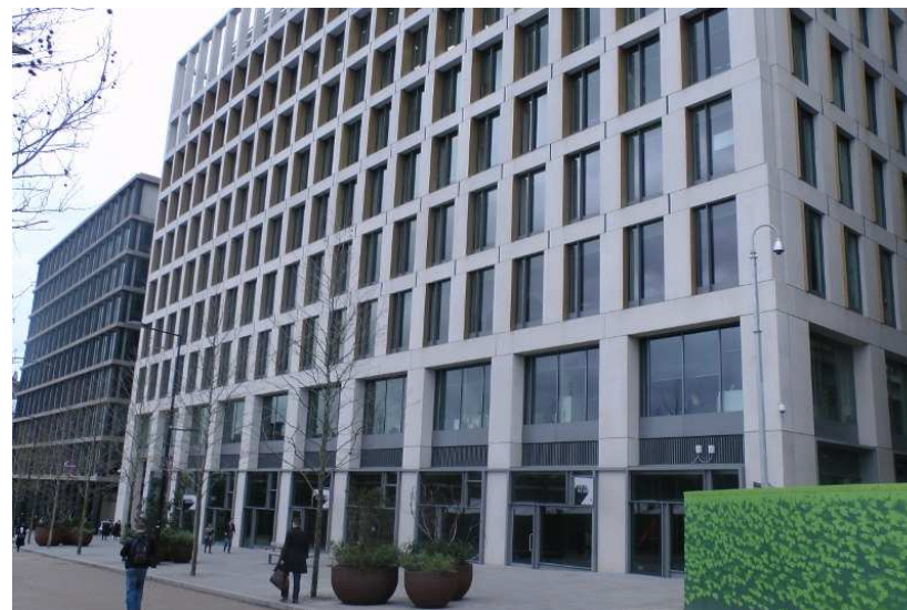
Townscape block at KingsCross Development
