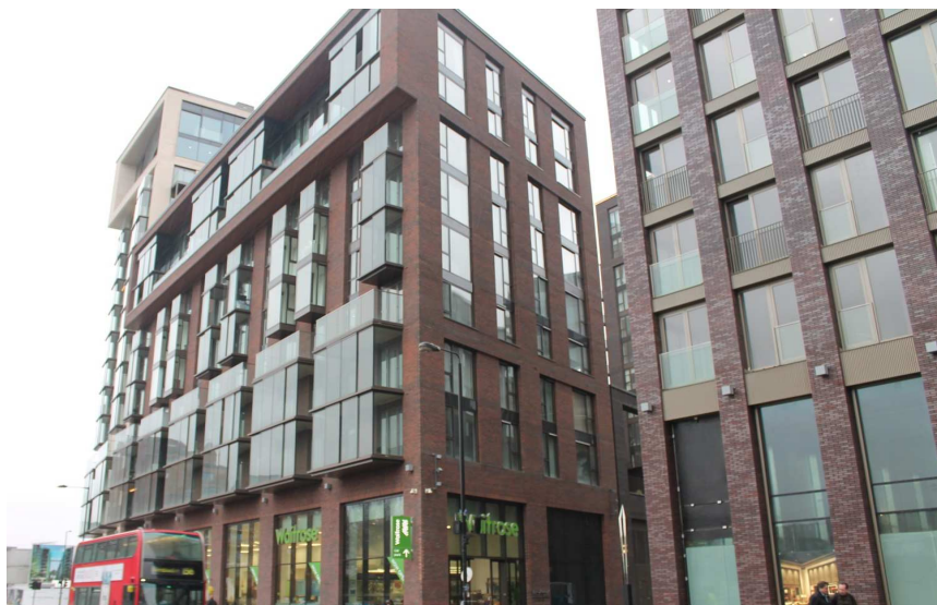
Townscape Block, Nine Elms, Battersea
