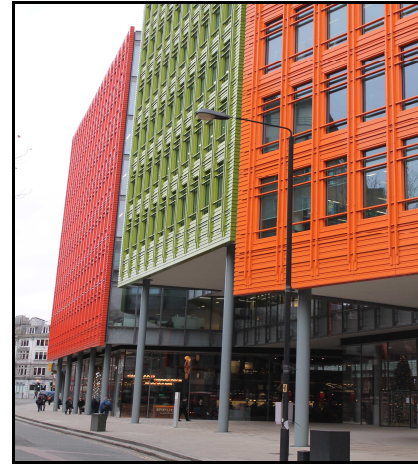
Good active street frontage
